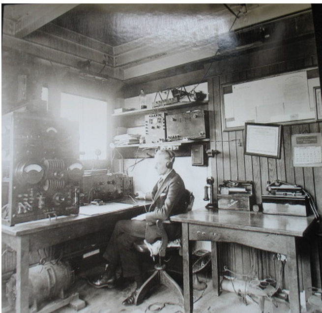
Figure 1 Wireless station on the roof of SCI's headquarters at 25 South Street [24]
